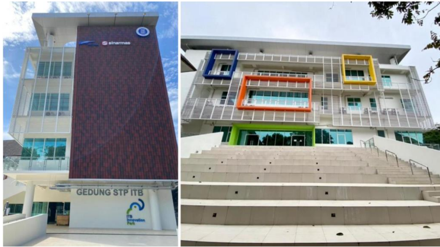
Gambar 6. Gedung Science and Techno Park.
